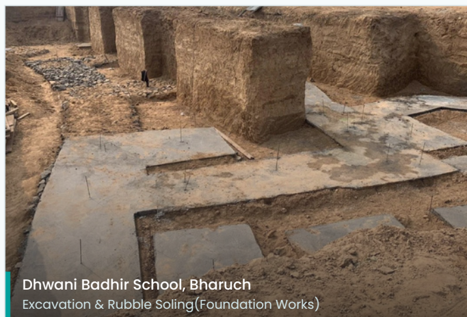
Dhwani Badhir School, Bharuch Excavation&RubbleSoling(Foundation Works)
